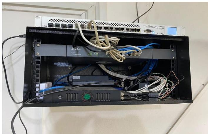
Figura 3 – Mikrotik Cloud Core Router CCR1036 e Switch 16 Portas Gigabit Tp-link Tl-sg1016d
